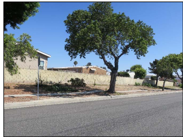
CMU perimeter wall at west side of property, view southeast.
