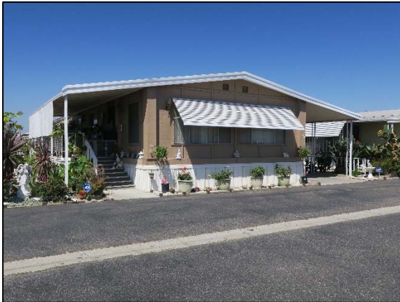
Example of typical older unit.
