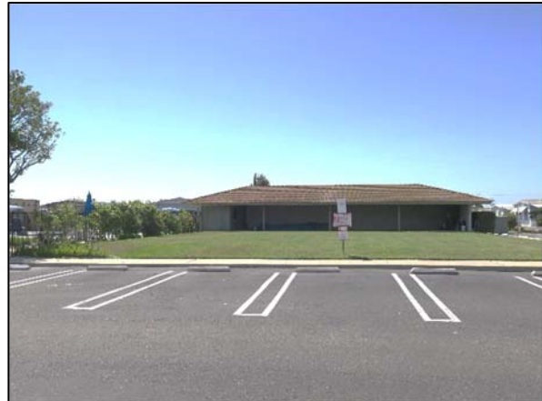
Open shed north of community building, view west.
