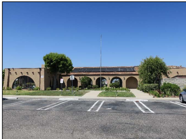
Community building south façade, view north.
