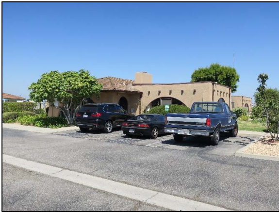
Overview of community building, view northeast.
