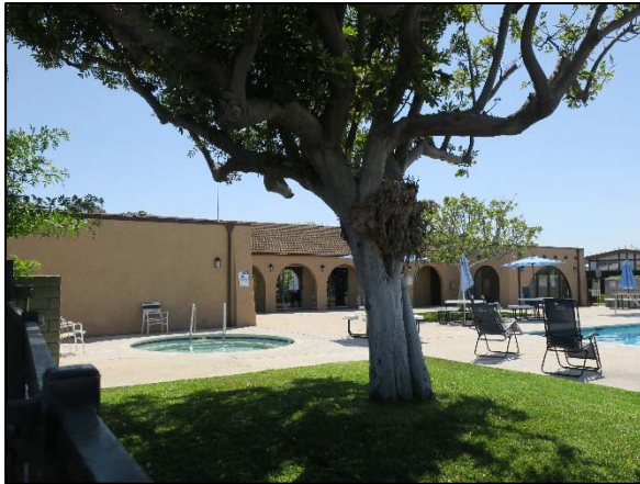
Community building north façade and portion of swimming pool, view southwest.
