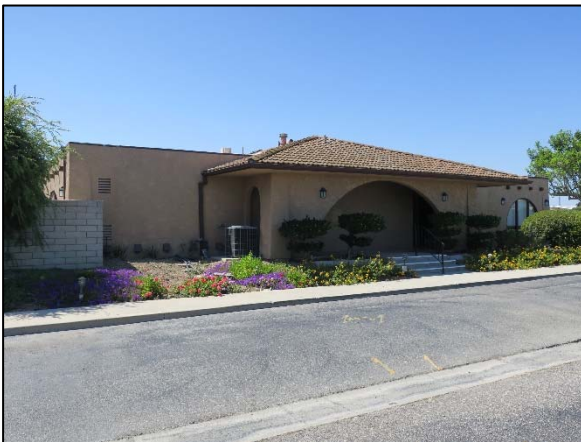
Community building east façade, view northwest.
